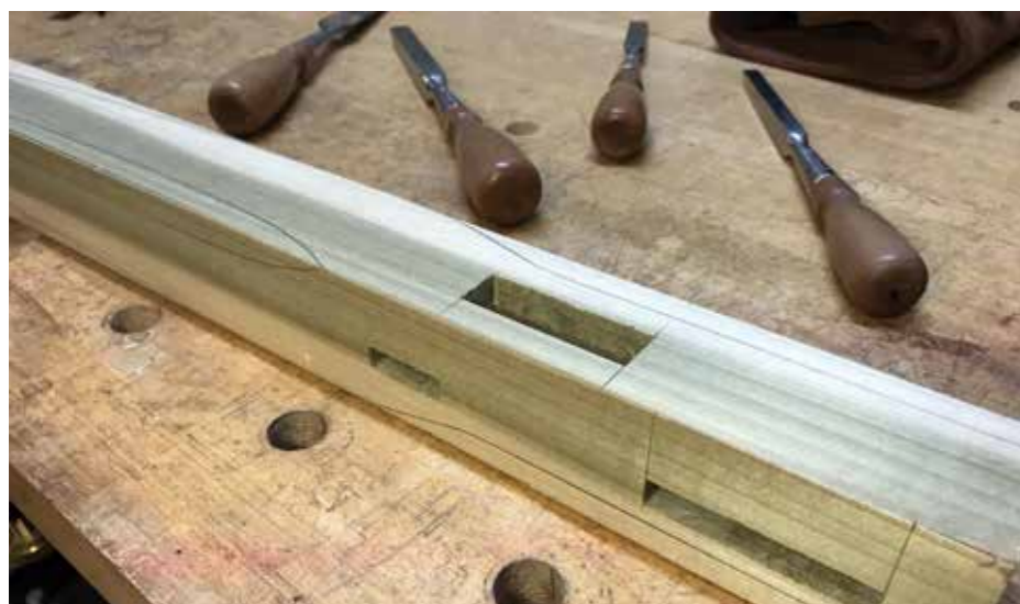
Be certain to lay out and excavate mortises before cutting to your pattern lines
